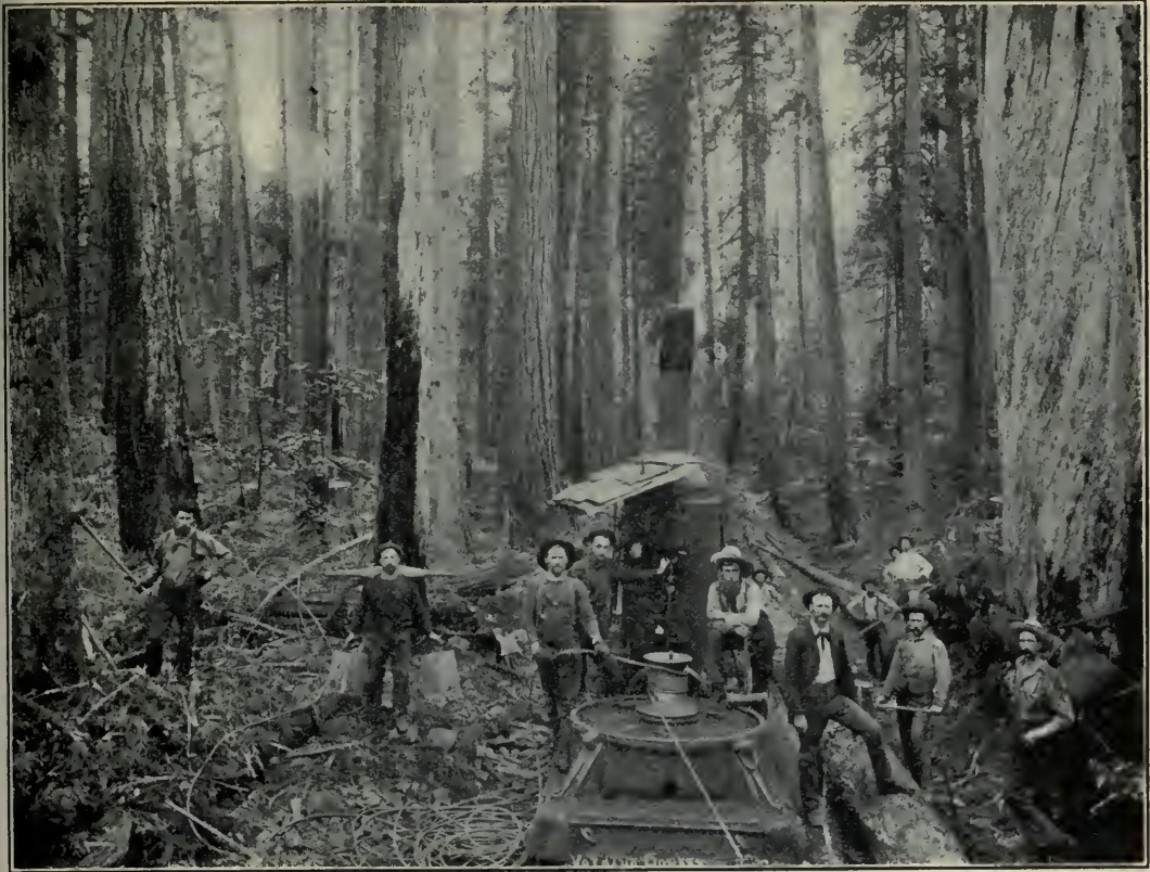
FIG. 296. — Lumbermen at work in the forest of western Washington. Note in the foreground the donkey engine used for drawing logs.
